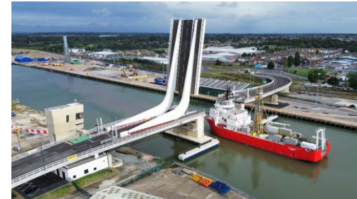
Lowestoft's Gull Wing Bridge
